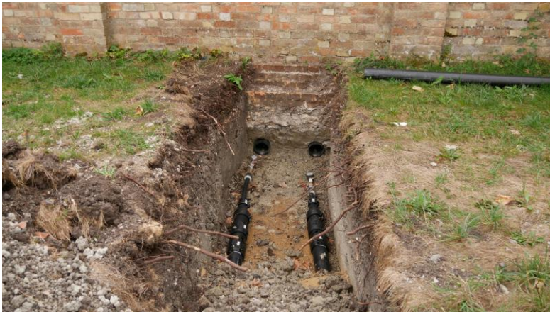
Ground source heating piping being installed at Wimpole, Cambridgeshire
